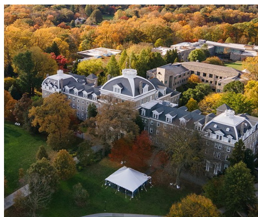
Aerial view of Parrish Hall.
